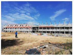
the 2. Floor they are preparing the roof. The steel work is done and soon the cement will put in.
