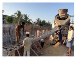
Now all the 4 walls are up, and few days ago a track has put the mud back. So the people can prepare the first roof. The level we are working on it is the underground level.
